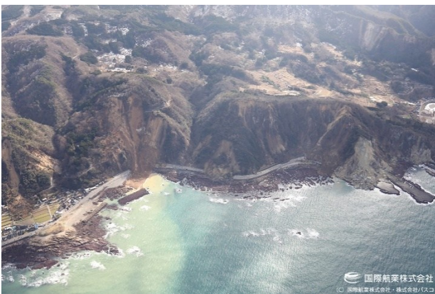
Figure 1, Landslide area on the northern coast of Noto Peninsula (January 2, 2024: Photo by Kokusai Kogyo).
