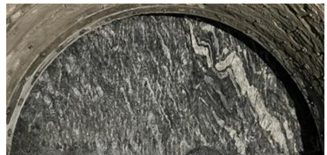
Figure 2, Fractured layer at 1+951.
