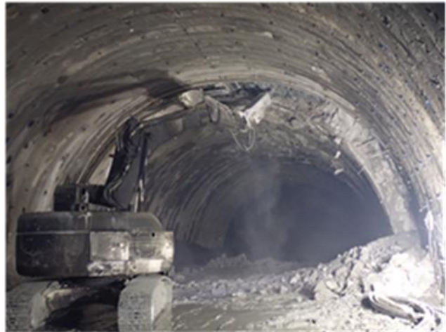
Figure 4 Re-excavation due to increased displacement.
