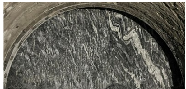
Figure 2, Fractured layer at 1+951.
