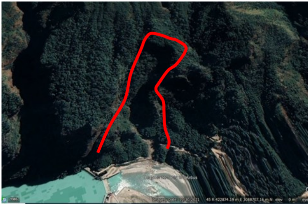
Figure 1, Scarp of paleo-landslide at the left abutment of damsite area.
