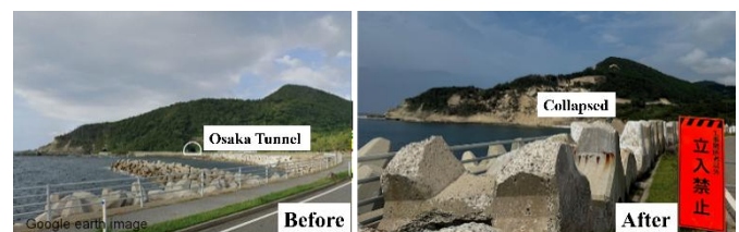
Figure 9, Collapsed Osaka tunnel before and after the 2024 Noto earthquake [date of photograph taken (after): August 4, 2024].
