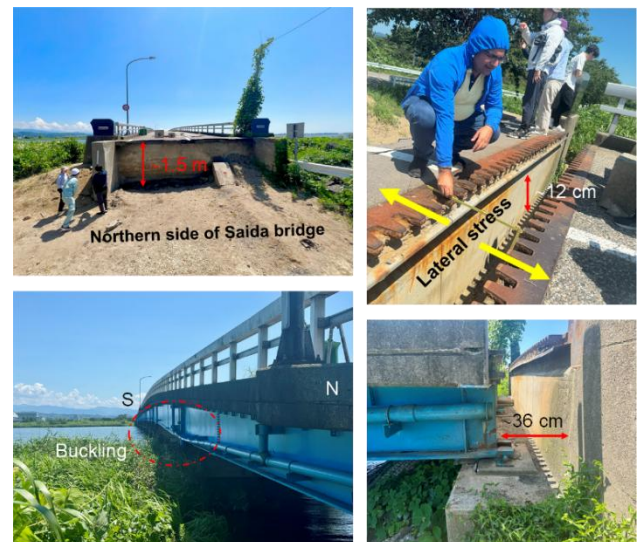
Figure 3, Damages in the Saida Bridge, Uchinada (Bridge offset vertically over tens of centimeters) (date of photographs taken: August 3, 2024).
