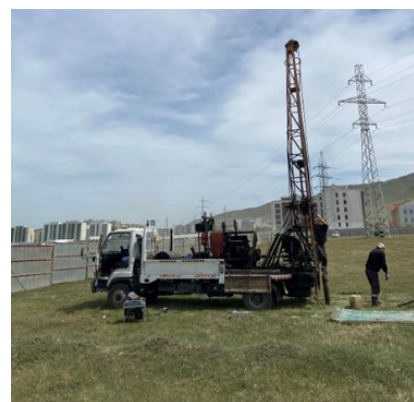
Figure 2, Drilling work at study area.
