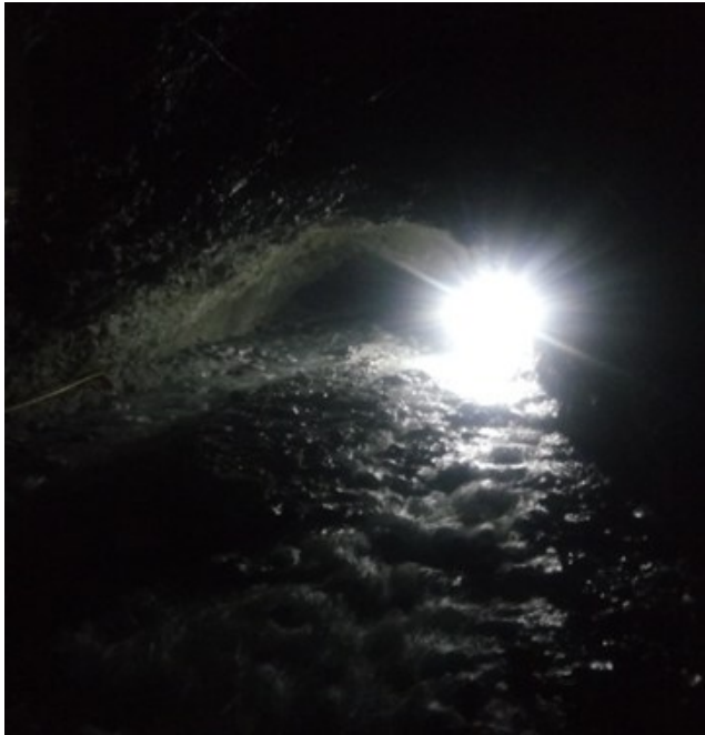
Figure 2, Debris Flow after over bursting Cavity.
