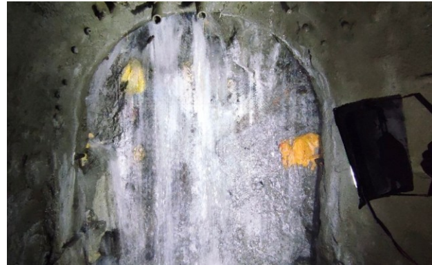
Figure 4, After Sealing of Face.
