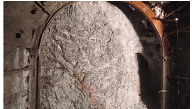
Figure 7, Rock Mass after Major cavity zone.
