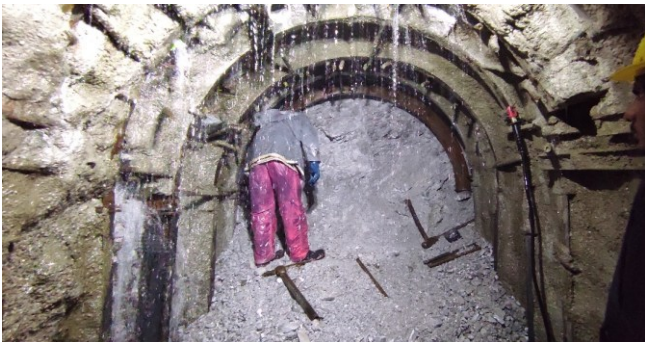
Figure 6, Heading and Benching -Excavation after Grouting.
