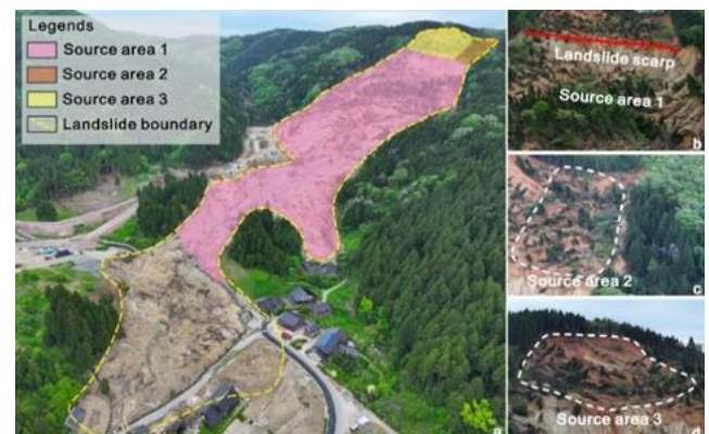
Figure 1, (a) Overview of Ichinose landslide; (b)–(d) Close-up Views of different locations of source area.
