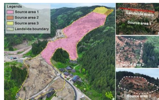
Figure 1, (a) Overview of Ichinose landslide; (b)–(d) Close-up Views of different locations of source area.
