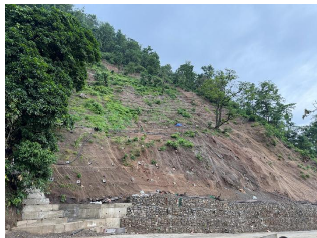
Figure 6, Jamunedanda slope after construction and completion of the mitigation works.
