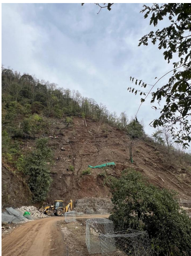
Figure 5, Jamunedanda slope before/during construction.
