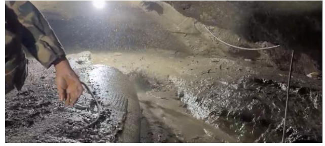
Figure 2, Water management and hydraulic debris-clearing works at Chilime
