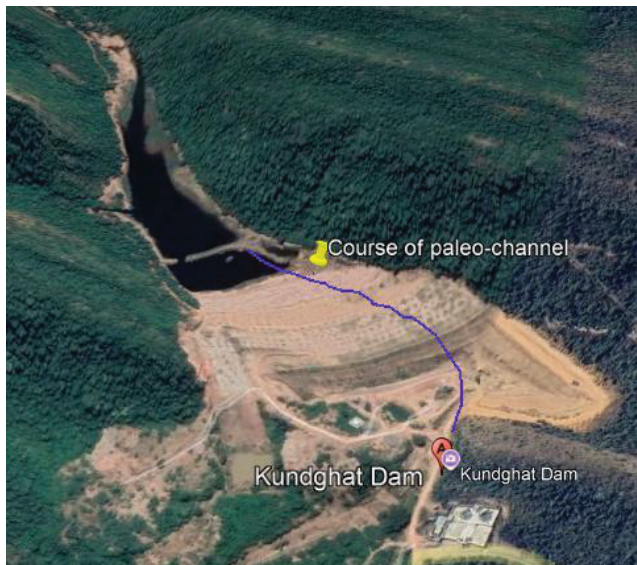
Figure 3, Course of the paleo-channel intercepted in excavations of the Cut-off-Trench (Source: GoogleEarth).
