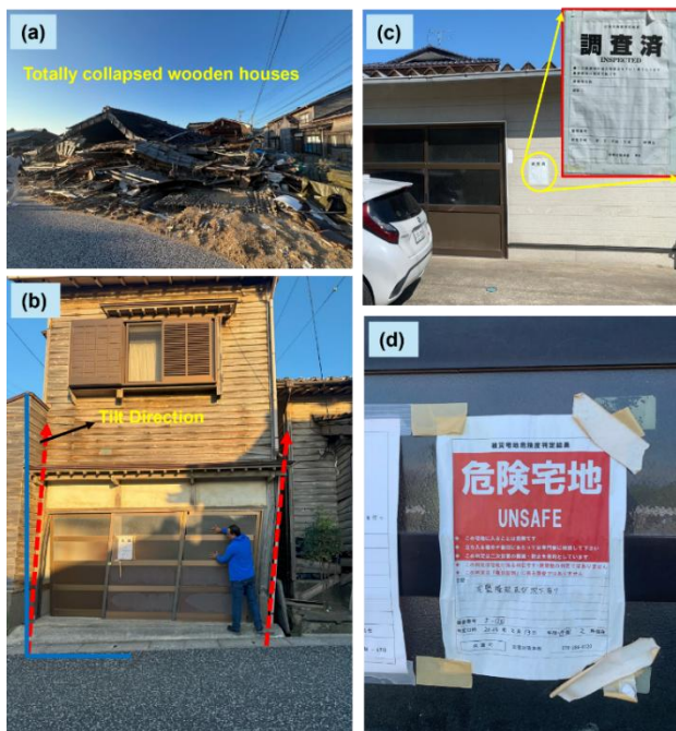
Figure 7, (a) Completely collapsed building along Wajima city; (b) tilted building; (c) building inspection certificate; and (d) inspection certificate attached to a building suffered with uplift and subsidence (date of photographs taken: August 3, 2024).
