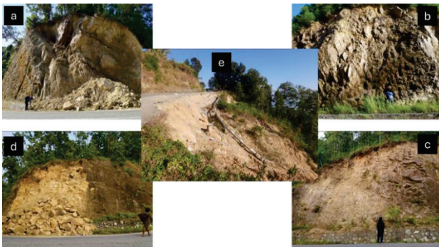
Figure 1, Representative slope conditions along the selected road section; a) Rockfall at Jitpur Bhanjyan, b) Joint sets at Taplakhar, c) Slope condition at Shikhar Kateri, d) Rock fall at Shikhar Kateri and e) Down slope failure at Bar Bhanjyan.
